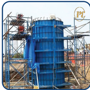
PIERS AND SHUUTER
